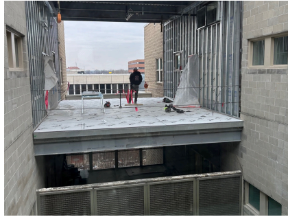
Construction began in 2025 to renovate the fourth floor of the Juvenile Justice Center.
